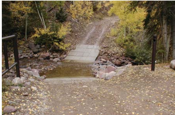
This ford on the headwaters of the Weber River has a firm rock bottom and the approaches have been hardened with concrete.
