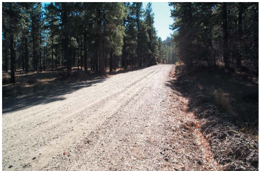
This forest road is located well away from water. Its gravel surface promotes drainage and lessens erosion. The road is crowned, so water drains away to both sides.
