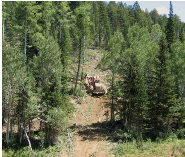
Skid trails such as this one in the Monte Cristo area need to be seeded and water-barred at the completion of the timber sale process.
