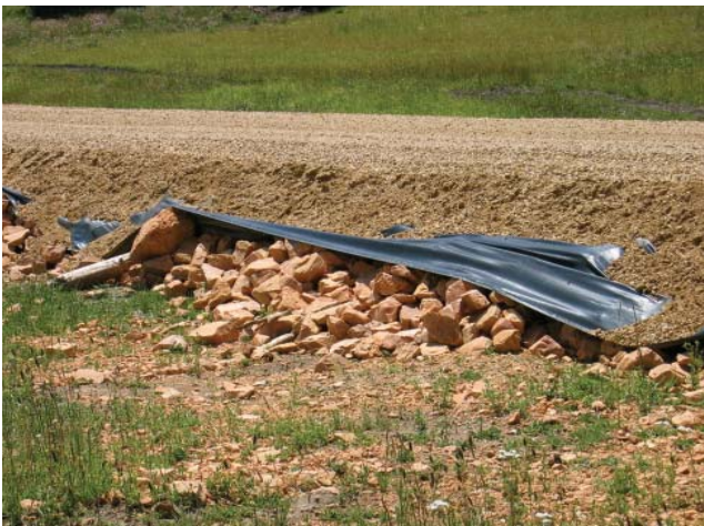
Geotextile is being used to strengthen this road through a wet area. Rock is laid on the wet surface, followed by geotextile and gravel on top.
